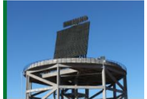
Fixed tower installation
