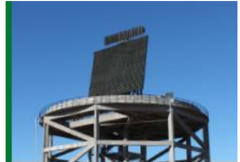
Fixed tower installation
